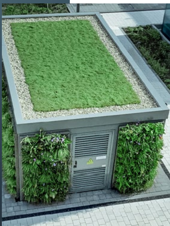
The first substation made of carbon concrete.
