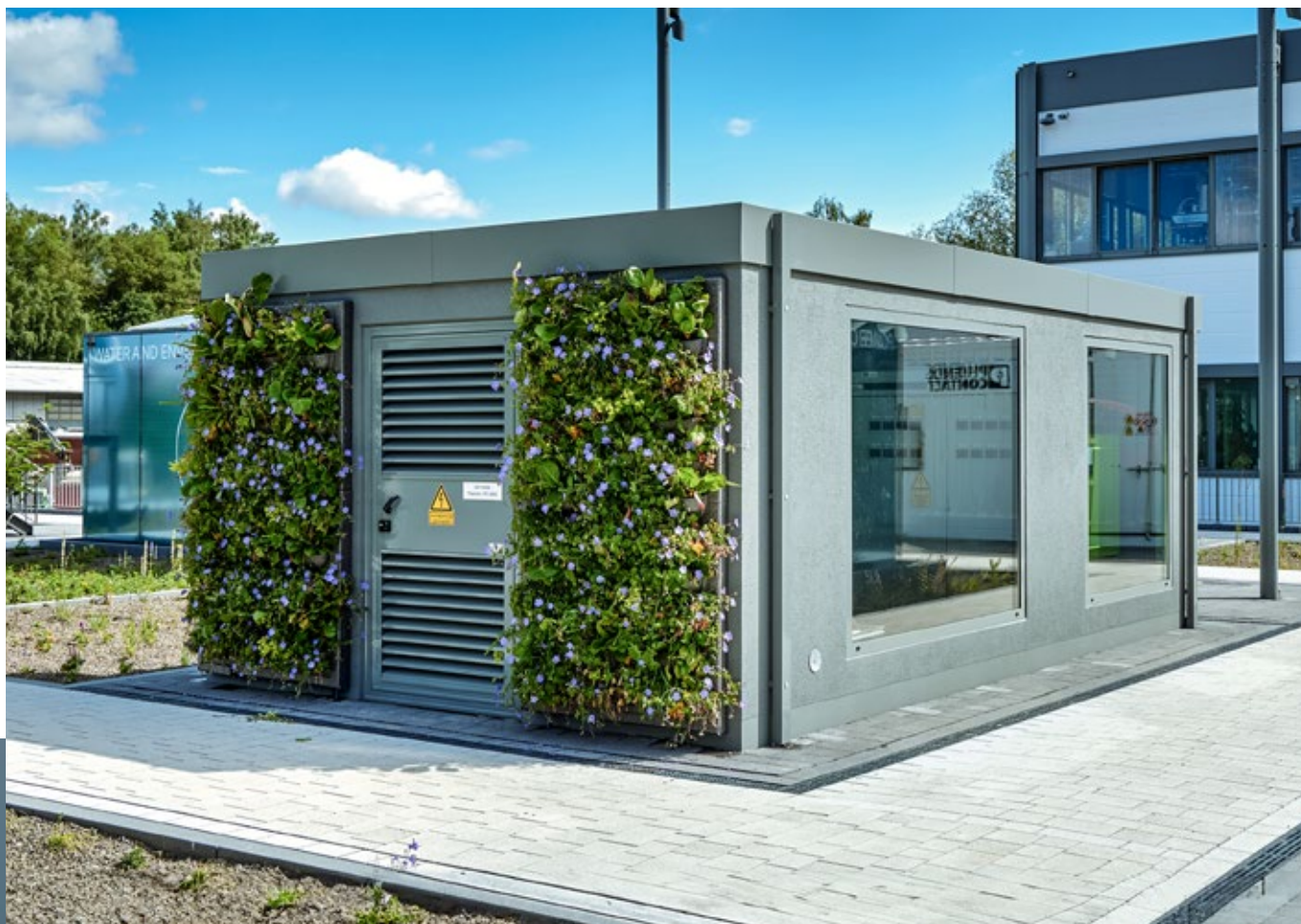
The first substation made of carbon concrete.
