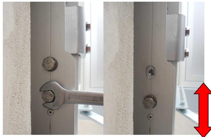
Fig. 2: Configuration of fastening screw union of the TAM3 door case
