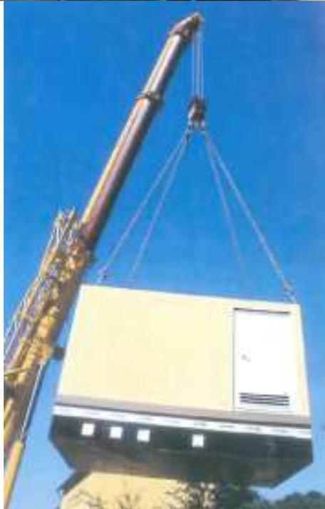
*Example of station suspension on the crane*
