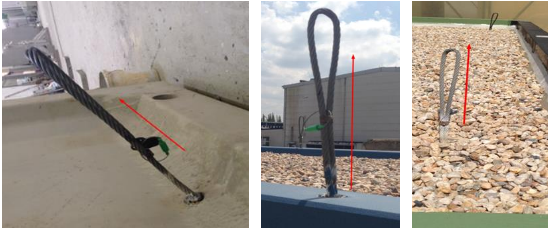
Fig. 24 Examples of permissible pull direction
