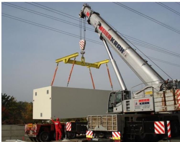
Fig. 28 Supporting beam (H-beam)
