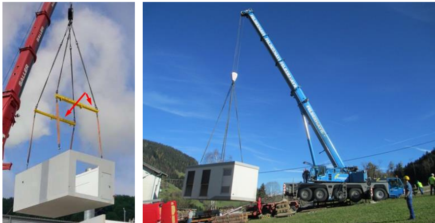
Fig. 19: Installation with and without a roof
