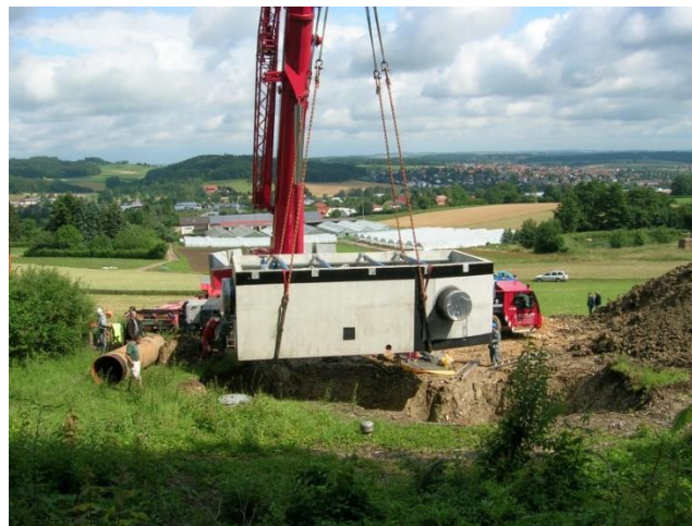
Fig. 23: Lifting the concrete cell with textile straps
