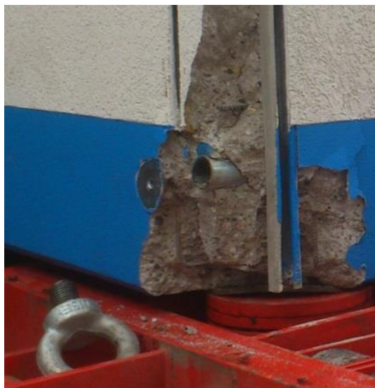
Fig. 8: Deformation caused by a prohibited lifting method
