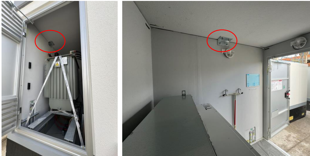
Fig. 22: Angles for securing during transport
